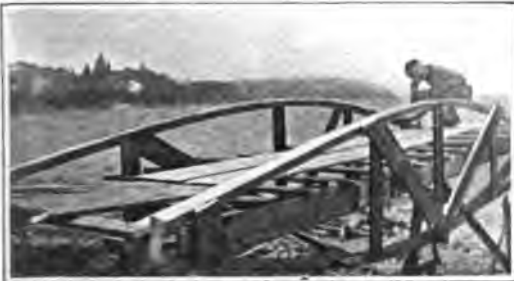
FIRST BOWSTRING SPAN IN POSITION
